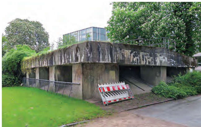
The unusual zerschellschicht (deflection or literally 'shattering' layer) of the Kaufmann command Bunker
